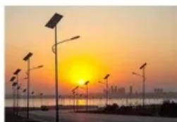
Solar Street Light
